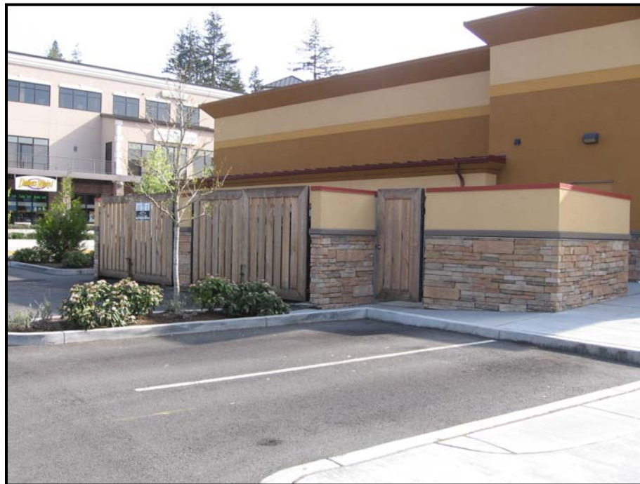
Service Areas Screened from Public View
